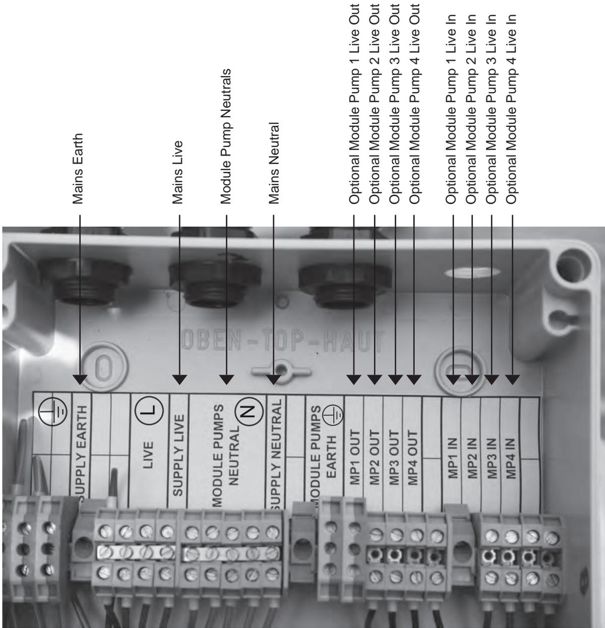
Connection 2: Inside Master PCB Box (top, right hand side of Master Module)
