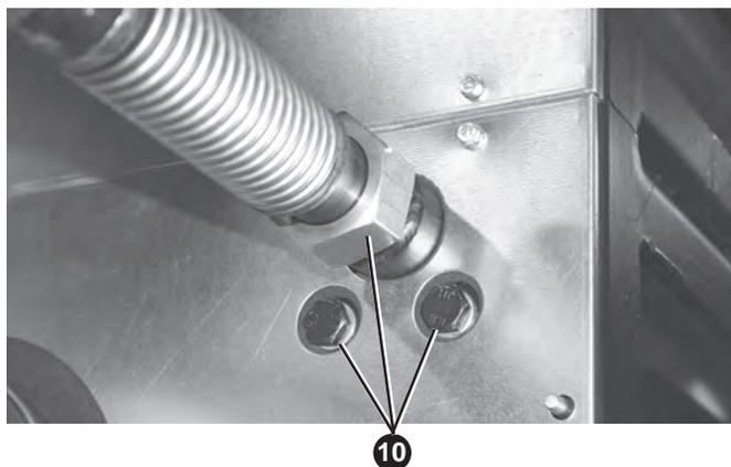
10. Remove the two fixing bolts at the gas connections and unscrew the gas union connections.
