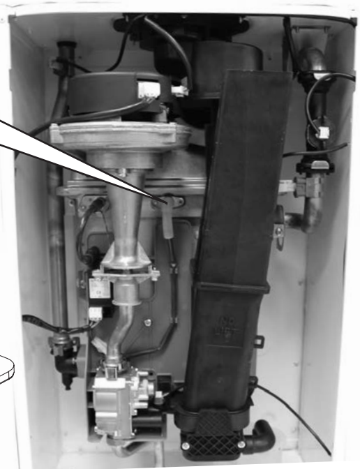
Flame Detection Electrode
