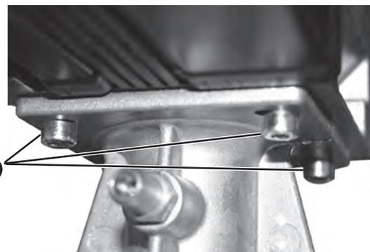
7. Withdraw the gas valve taking care to retain the inlet and outlet 'O' rings.
