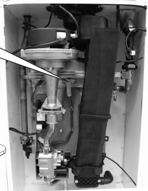
Flame Detection Electrode
