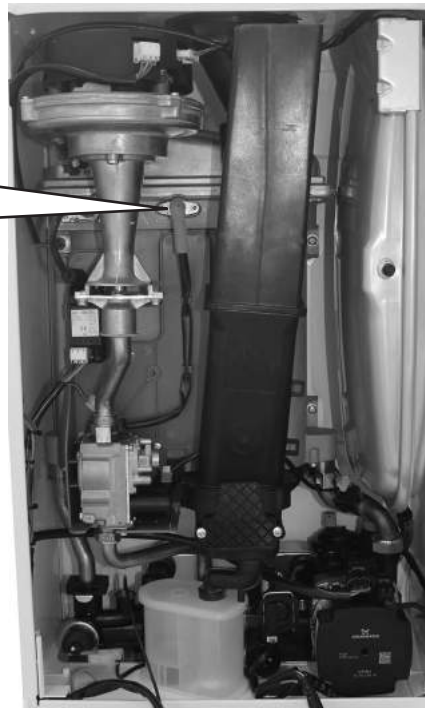
Flame Detection Electrode
