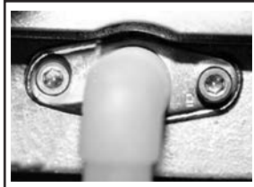
Flame Detection Electrode
